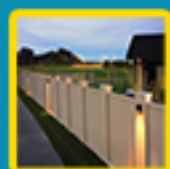
Fully Compounded Wall
